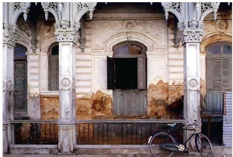
Figure 5: Unlike lime plaster, the Portland cement is not compatible with the masonry substrate, leading to water damage to the structural walls. (Aga Khan Trust for Culture 1993).
